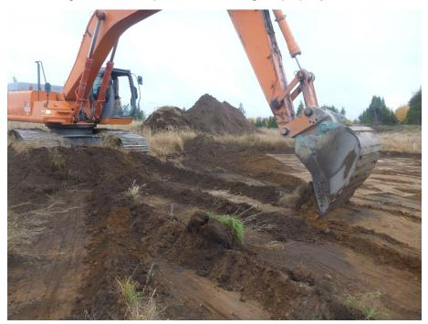
Image 4: Excavator conducting mechanical topsoil removal view northeast.
