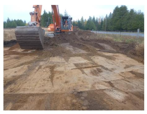
Image 3: Excavator conducting mechanical topsoil removal along the property fenceline, view southwest.
